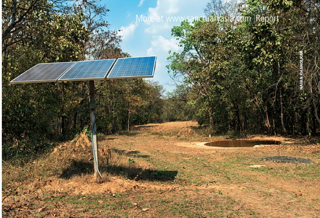
Solar-powered freshwater borewells have been installed at strategic points by the Forest Department to replenish small waterbodies, streams and artificially-created waterholes.
